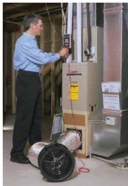
The Duct Blaster® can measure the total amount of air moving through the air handler.
